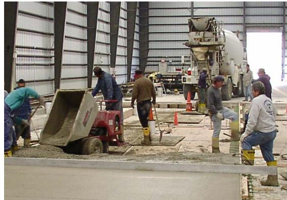
FIGURE 32. POWER BUGGY USED AT THE NAPTF TO TRANSPORT FRESH CONCRETE FROM MIXER
