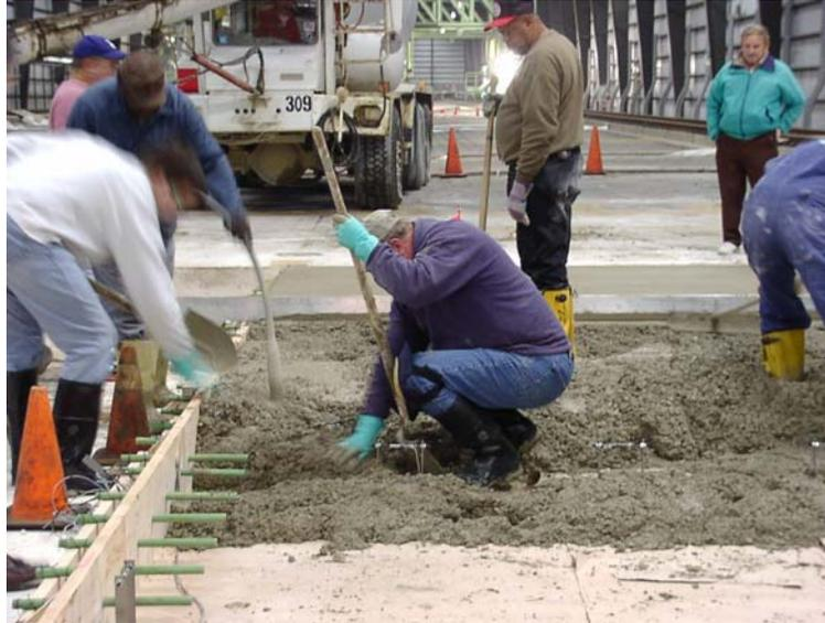
FIGURE 35. VIBRATING CONCRETE DURING PLACEMENT OF TEST STRIPS AT THE NAPTF
